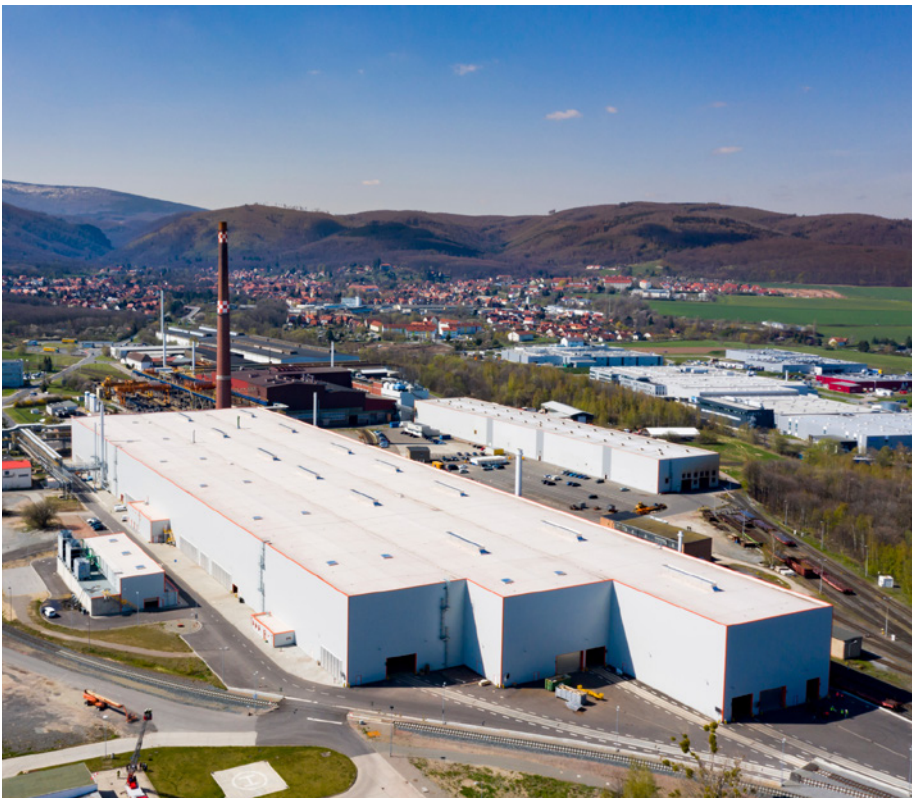
The new heat-treatment facilities at Ilsenburger Grobblech are accommodated in a complex of three new buildings covering an area of 31.290 square metres (Picture: Ilsenburger Grobblech GmbH)
